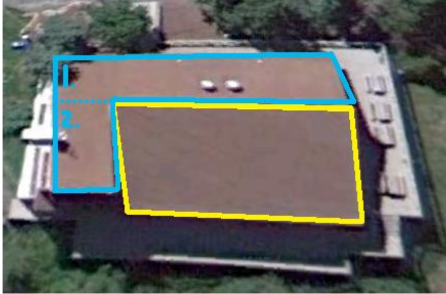
Figure D.1: Aerial view of CamelTop, showing three separate roof sections: A (yellow), B1 and B2 (blue) (Google Earth, 2011). Only south-facing sections are being considered for optimal PV placement.
